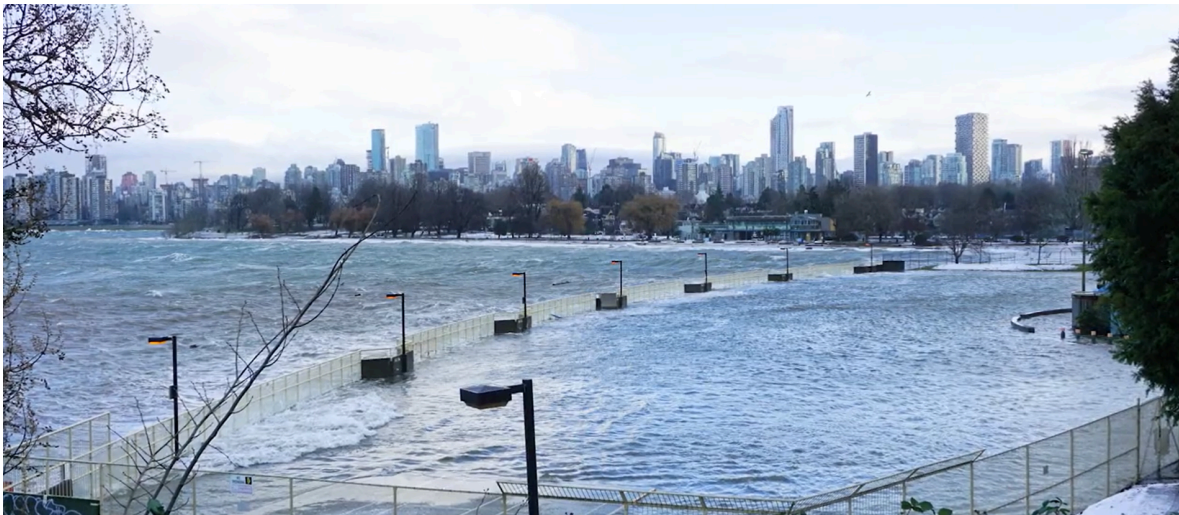
Figure 8. King tides in winter storms have caused significant structural damage to Kitsilano Outdoor Pool (Catherine Urquhart, 2022)
